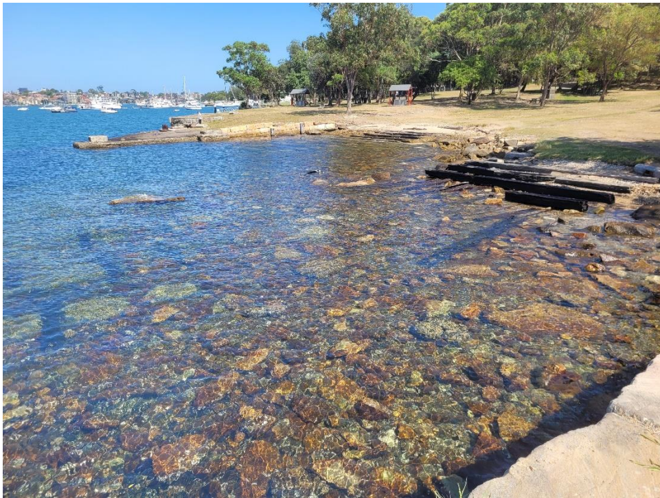
Figure 3: Significant fabric of the slipways established by Atlas Engineering remains as do other items associated with ship construction such as the concrete blocks and other items seen on the foreshore beyond the western slipway. A great deal of debris has found its way on to the slipways.
