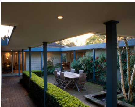
Above: Eastern elevation from Tیره Avenue, 1961. Photo: Max Dupain, courtesy SLNSW.
