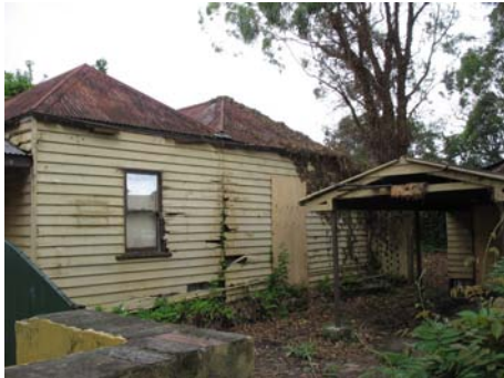
11 Mark St prior to demolition with its double pitch roof
