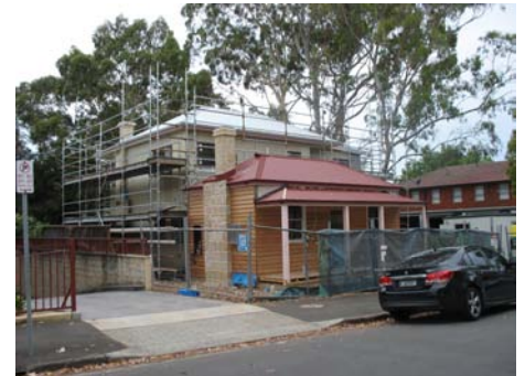
11 Mark St under construction with the rebuilt cottage element in front
