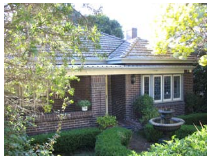
21 Abigail St – its neighbour demolished
