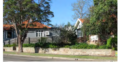
The restored front fence at 38 Ryde Rd
