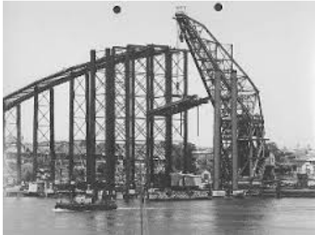
Gladesville Bridge Under construction
