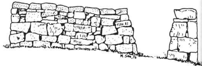
Early dry stone wall, at the back of Herberton Avenue, built of roughly shaped stones with rectangular capping stones. Slightly wider at base for stability
