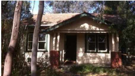
The house in East Kew demolished
