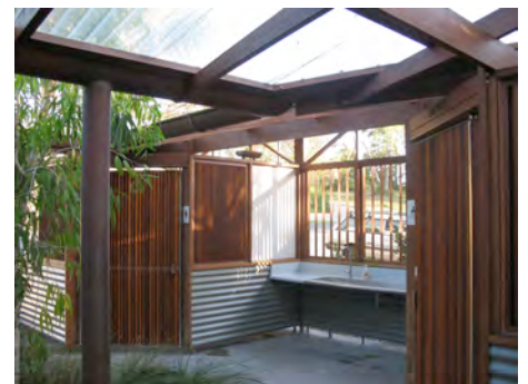
Toilet block at Middle Head – Sydney Harbour Federation Trust
