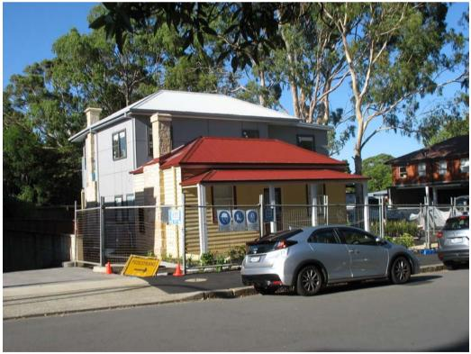
The restoration of the existing cottage paid little attention to existing details such as the profiles of the weatherboards or the colours. Unfortunately CAP's prediction that the scale of the new rear section would overwhelm the existing cottage was totally vindicated. **But wait – there's more!**
