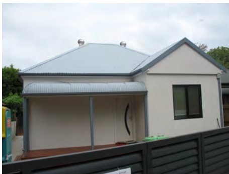
Ryde Road house after
