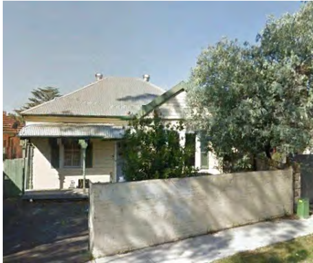
83 Ryde Road before (Google street view)
