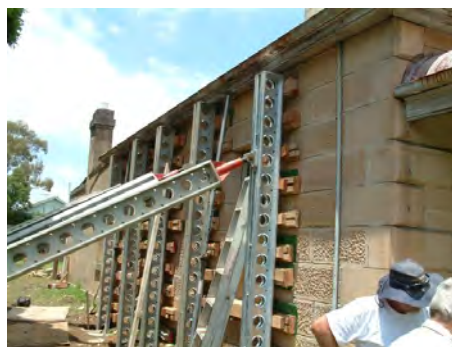
59 Pittwater Rd rectification work
