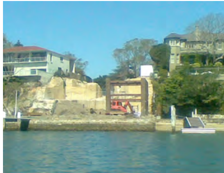
Sandstone excavation at The Point Road as seen from the water
